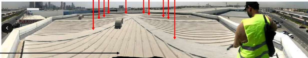
Full Panoramic View of this roof taken from this point.
